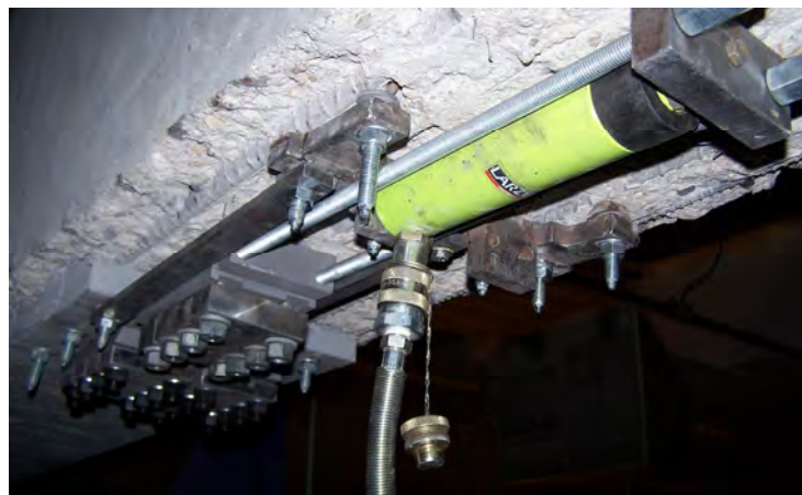
Fig. 15. Active anchorage
