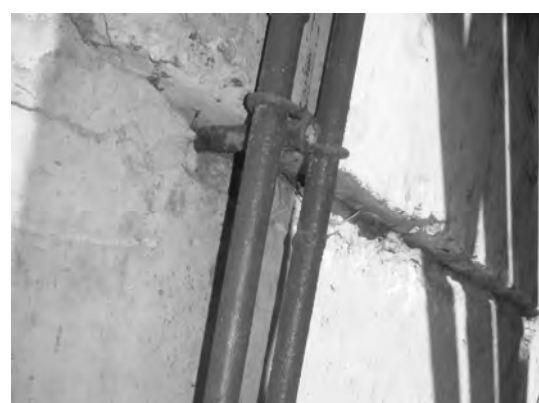
Photo 4. The state of the foundation wall blocks by axis "A" between axes "2" ... "3". Deviation from vertical, moving units by seams
