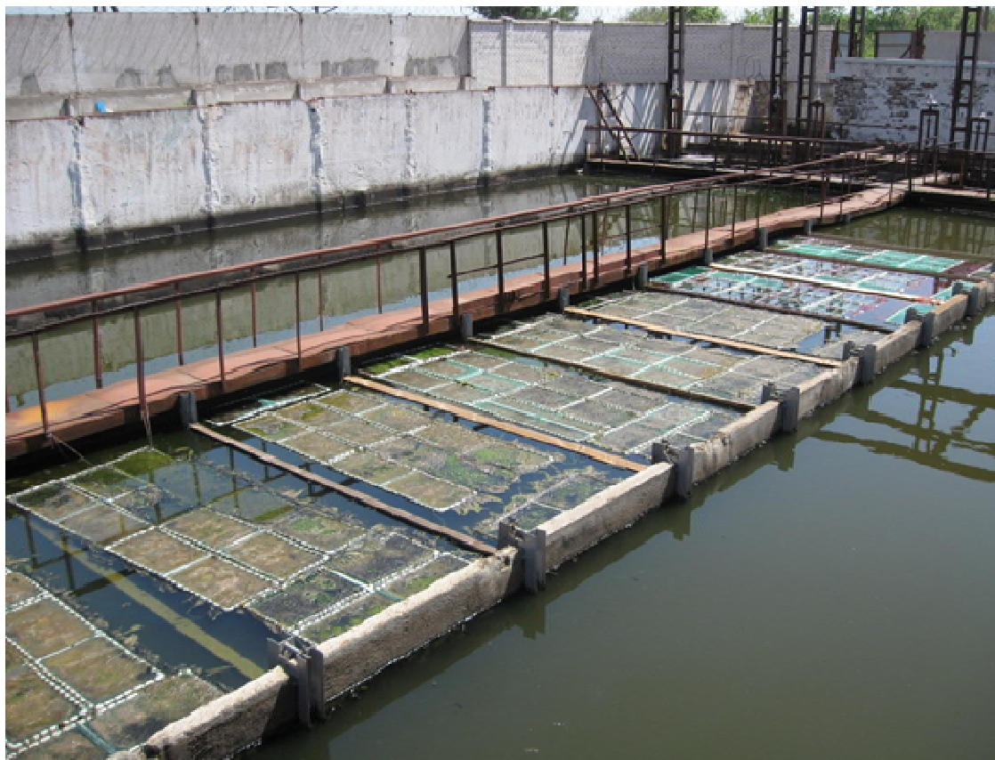
Fig. Seventy-six mounted rafts with fibrous carrier “VIYA” installed in one experimental storm treatment facility (STF) tank No. 54 of the plant “Motor Sich JSC”
