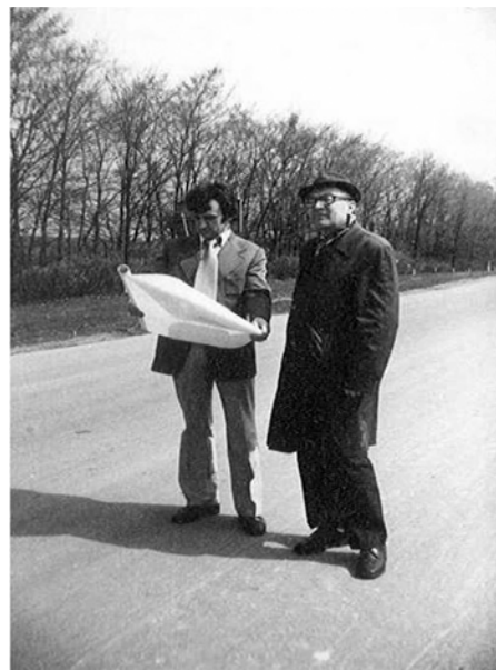
Fig. 4. Professor Rudnytskyi and assistant Habel at the sign construction site. (from the author’s private records)
