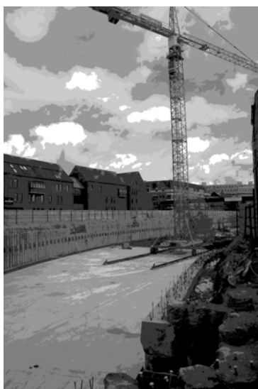
Fig. 2. Rebuilding of Thomas B. Thriges Street, Odense; photo by O. Gazińska, 14.07.2015
