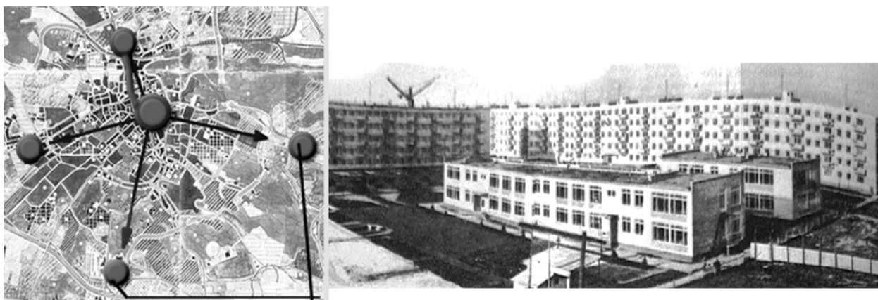
Fig. 5. Project of development of the polycentric system of the city centre of Lviv, 1970 (authors J. Novakivsky, P. Myh, A. Petrova, A. Rudnytskyi)
