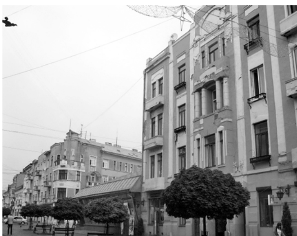
Fig. 7. The buildings of Kobylianska Street in Chernivtsy, Ukraine. The current situation. Photo [13]
