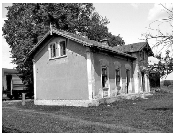
Fig. 10. The railway station of Petrivtsi, Bukovyna. Author's Photo, 2006
