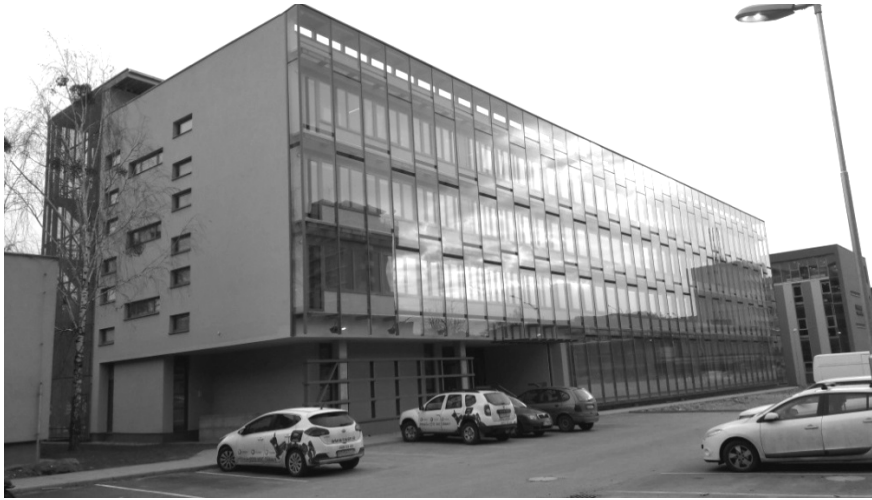
Fig. 1. Front view (WEST) of TECHNIKOM (Science & Technology Park) building
