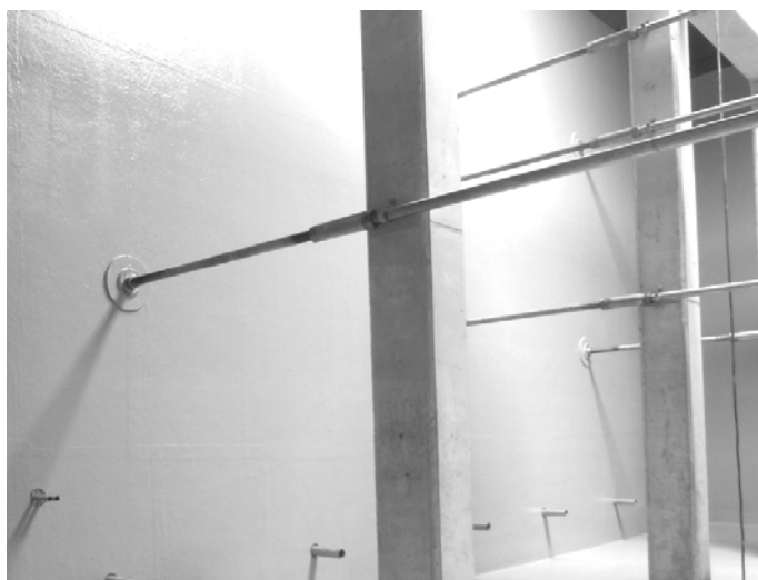
Fig. 6. Tie-bars installed and supported on the inner columns
