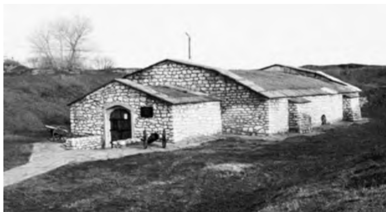
Fig. 7. Actual condition of St. Volodymyr bastion and powder magazine inside, Tiraspol. Author's photo
