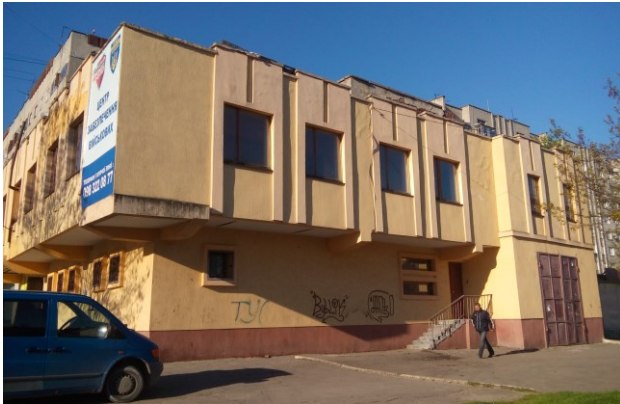
Fig. 6. The existing exterior of the building of the household service center in Riasne-1
