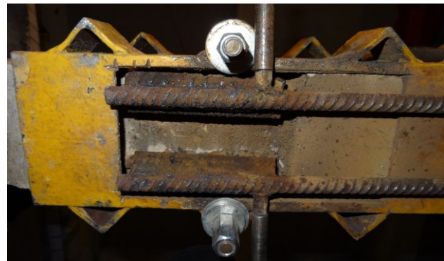
Fig. 3. The beam strengthened with prestressed reinforcing bars
