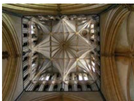
Fig.37. Star-shaped vault, Lincoln's Cathedral, England [16]
