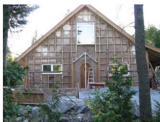
Pic.7. Restoration of a rain-washed facade.
