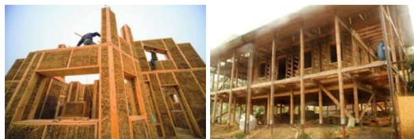
Pic. 1-2. village Hotyanovka, Kiev region. The biggest house made of straw in Ukraine
