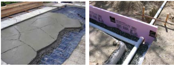
Pic. 16-17. Laying the foundation
