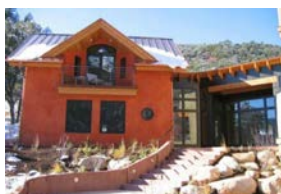
Pic. 13. Stable and energy-efficient homes from straw block
