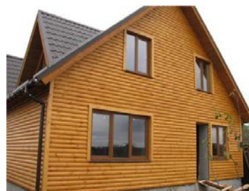
Pic. 41. House of straw in Kiev region. Construction of the house was handled by Valery Gomenyuk and his team
