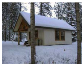
Pic. 29. Final look of the house
