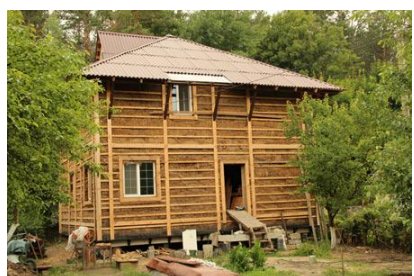
Pic. 37. House of strawbales near Kiev. The owner of the house and the author of the project is Artem Domashenko
