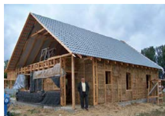
Pic. 38. A frame house with straw insulation under Poltava. Andrei Konyuk, Radion Khovanets, Oleg Ivanenko worked on project of the house and its construction.
