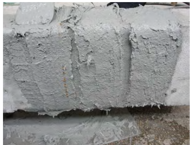
Fig. 3. Causing FRCM system on the beam
