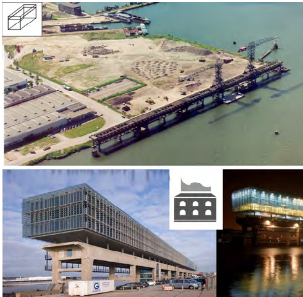
Fig. 2. Kraanspoor - very light , glass , three-story office building constructed on the existing concrete unloading board. This platform is built in 1952 , length of 270 m, a height of 13.5 m and a width of 8.7 m - a monument of industrial design
