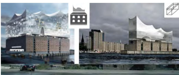
Fig. 3 Renovation of port dock under Philharmonic, red brick building , built in 1963 by Werner Kallmorgenom. Contrast of glass and industrial design
