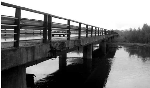
Fig. 6. General view on Baranów Bridge
