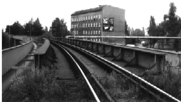
Fig. 1. Top view of the railway bridge and multi-family residential house
