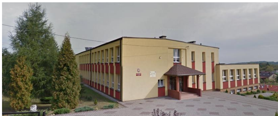
Fig. 7. Entrance elevation of monitored building
