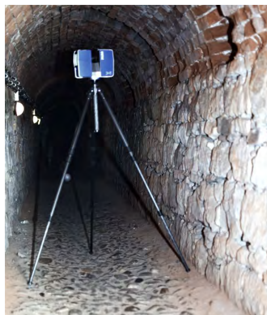
Fig. 7. Faro focus3D x 330 in the underground sidewalk
