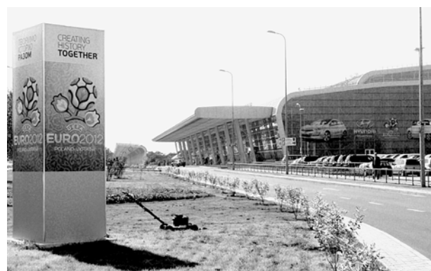
Fig. 21. New airport terminal. (© Bohdan Posatskyy, 2012)
