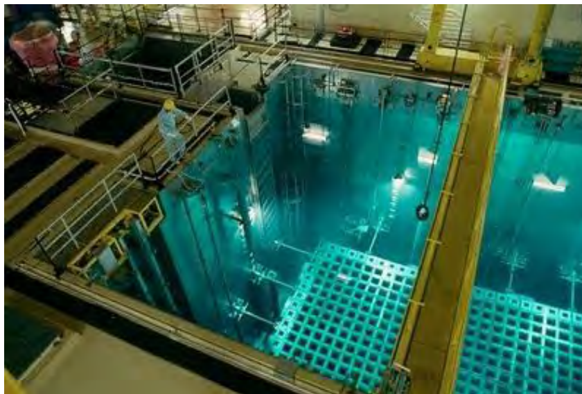
Fig. 1. Pool for storage of spent nuclear fuel at NPP
