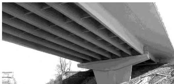
Fig.2 Appearance of road bridge after reconstruction
