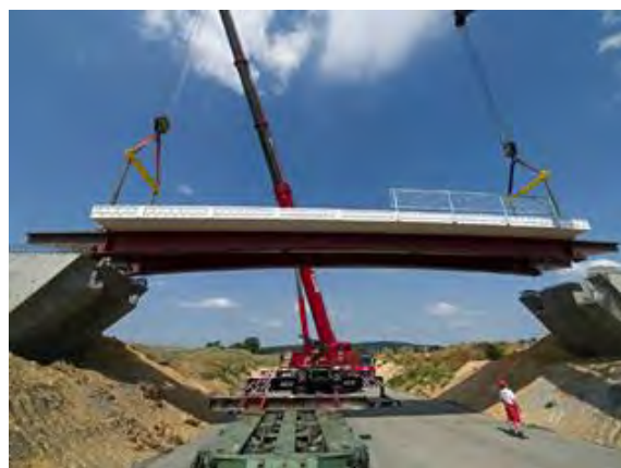
Fig.3 First long plastics road bridge in Germany
