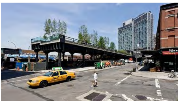
Fig.6 The High - New York City linear park built on elevated former New York Central Railroad spur
