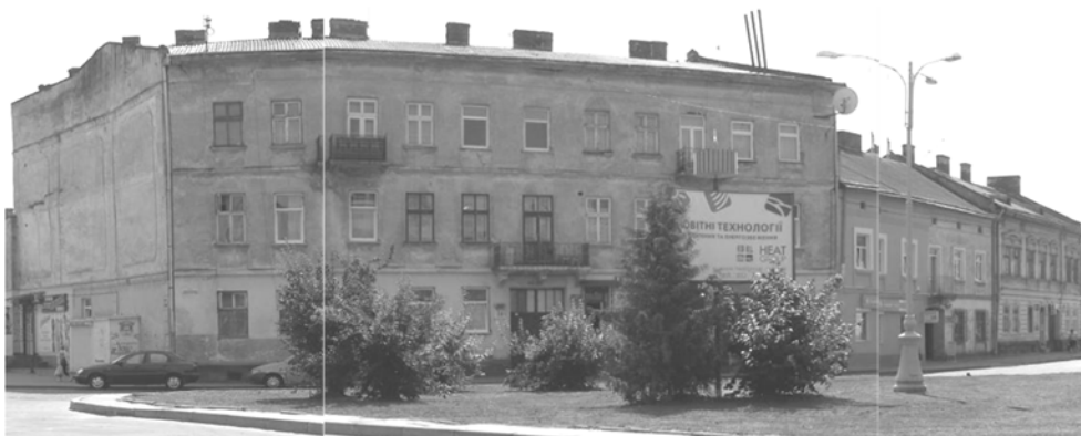
Fig. 1. A group of three residential buildings № 34, 32, 30 (from left - to right) on Dzherel'na street in Lviv
