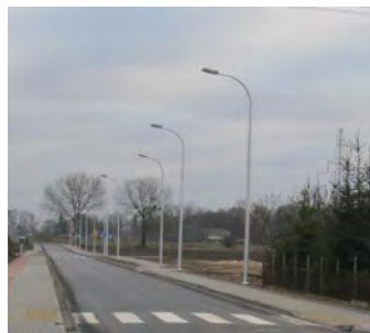
Fig. 2. Pavement view during tests in December 2011
