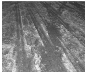
Fig. 3. Pavement view during tests in February 2012
