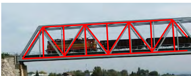
Fig. 2. Proposal of the computational model-plane truss [1]
