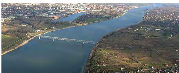
Fig. 1. The railway bridge over the river Danube at Komárno [1]
