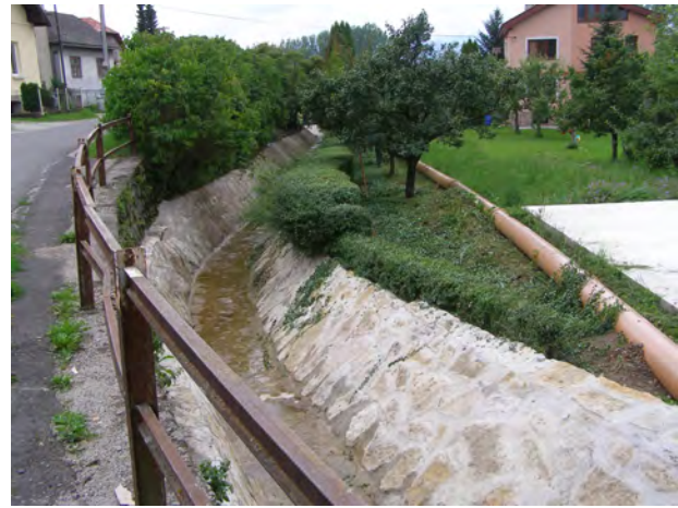
Fig. 8. Creek in Vydrník village – adjusted state
