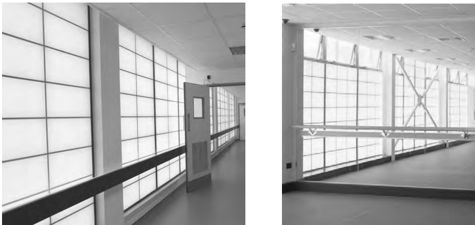
Fig. 5, 6. Examples of the use of aerogel panels (hall and gym) [9]
