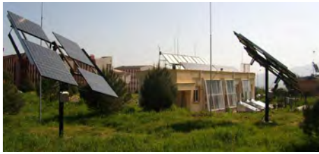
Fig. 1. Photovoltaics at Clean Energy House (CEH)
