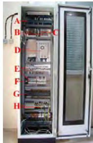
Fig. 2. DC power distribution panel [2], [3].
