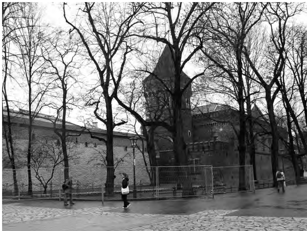
Fig. 12. A section of defensive walls after conservation works and of the covered passageway made of broken limestone in the pavement; a culvert of dolomite slabs, photo by. H. Rojkowska.
