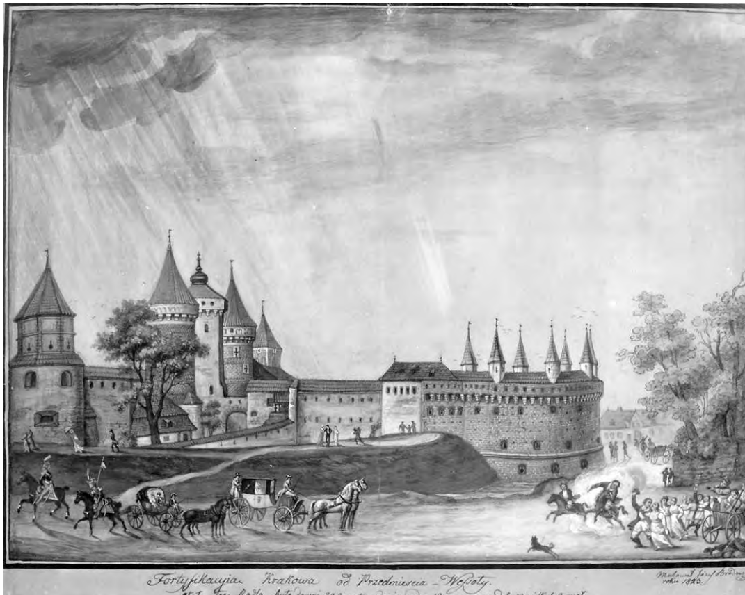
Fig. 1. Józef Brodowski, a view of the defensive walls from north-east before their removal, 1823
