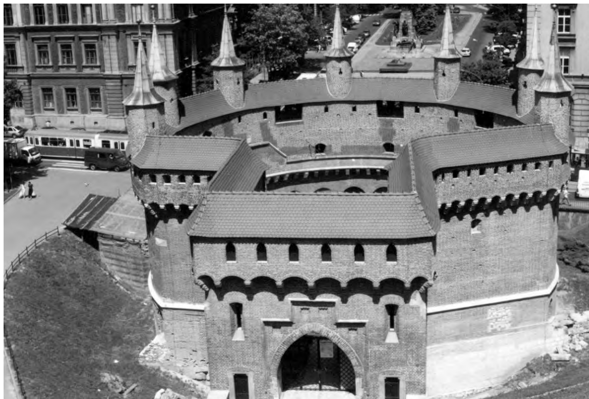
Fig. 6. Barbican under conservation works in 2001, photo by H. Rojkowska
