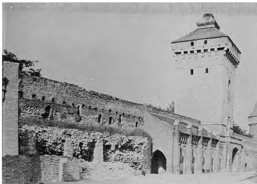
Fig. 9. Western curtain wall from the south during restoration works in 1897., L. P. Jouedrau, Paris, around 1897.
