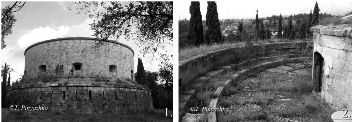
Fig. 14. Verona: 1 – the small maximilian tower nr. III; 2 – view from the roof terrace of the small maximilian tower nr. I. Photo's 2011
